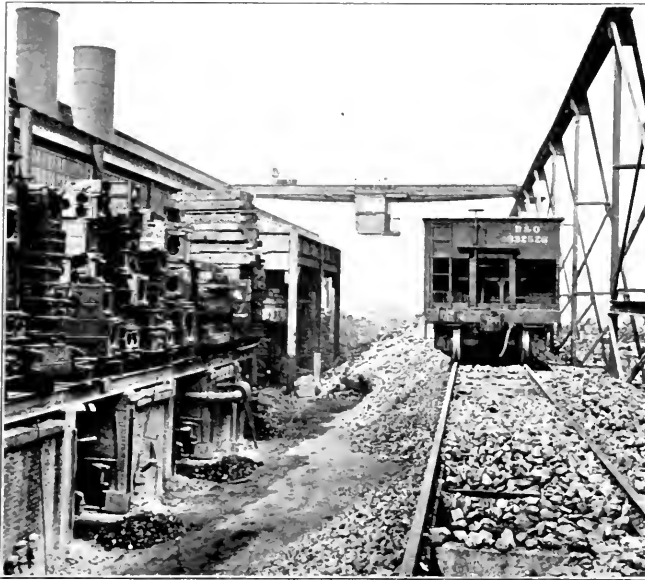
FIG. 5. TRESTLE AND OVERHEAD CRANE USED IN MATERIALS HANDLING
